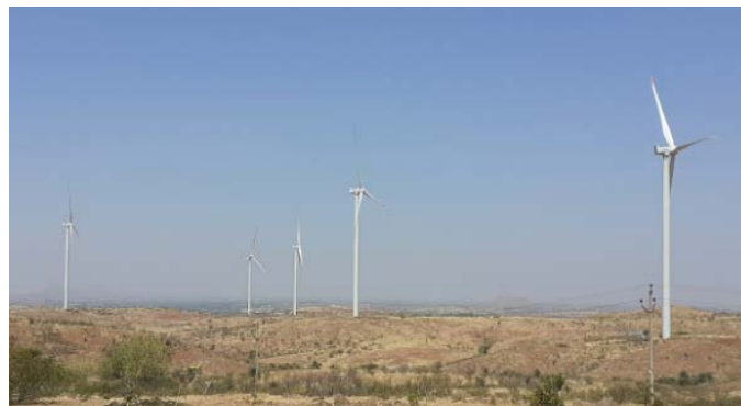
Figure 2: Installed wind turbines at the studied location
